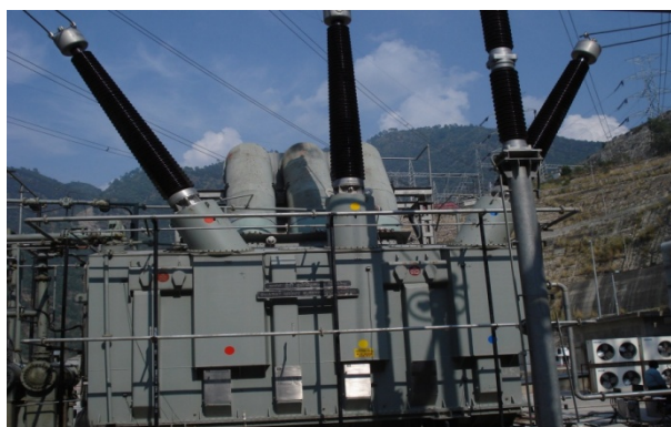
Fig.1 Generator Transformer of Koteshwar HEP
